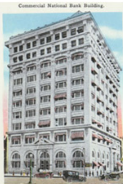
Commercial National Bank Building.
