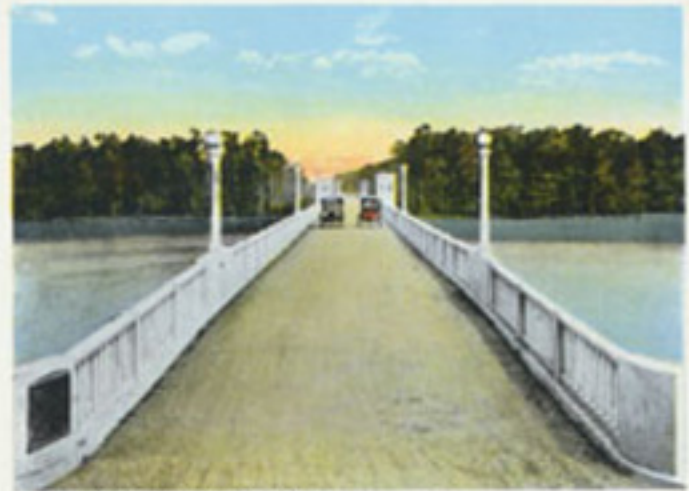
BRIDGE ACROSS CALCASIEU RIVER.
